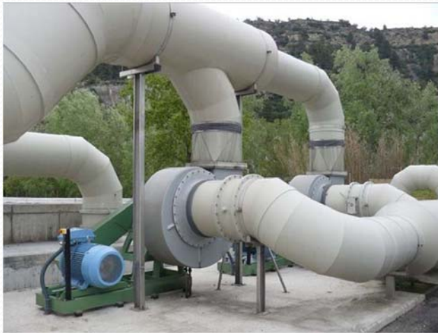
Before pilot plant installation
