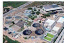
Waste Water Camp Tarragona WWTP
